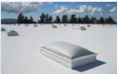
Roof with white TPO coating
