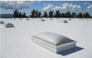
Roof with white TPO coating
